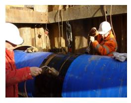
**5.** Check edges of sleeve to ensure mastic "wetting out". Use a roller if needed.
