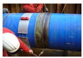
Clean joint with power wire brush to ST3 minimum & lightly abrade adjacent coating. Degrease using cleaner and clean rags. Preheat pipe to 70°C (temp. sticks will be provided).
