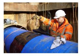
**3.** Heat the underside of the closure strip with 4 passes of the propane torch and place over the overlap. Install the closure strip properly before heating the rest of the sleeve.
