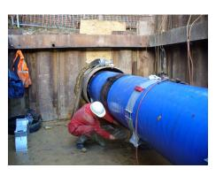
2. Wrap sleeve around the pipe joint, starting at 11 o'clock and passing the sleeve underneath and back over the top for the overlap.
