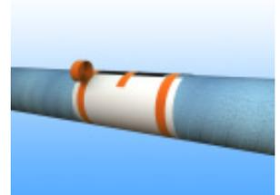
3. Check that the mould sits firmly around the pipe circumference and make sure that there is no bend in the area of the filling slot. For pipe diameters of DN 100 to DN 200, two moulds must be prepared before mixing the mortar.
