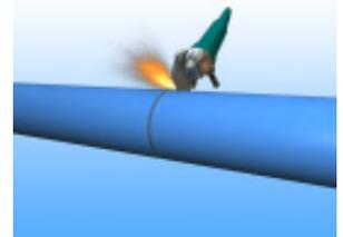
To remove the fibre cement coating, e.g. at the end of shortened pipes, or in order to apply saddle fittings on the polyethylene coating, make incisions into the FCM coating around the pipe circumference and along the length to be removed.
